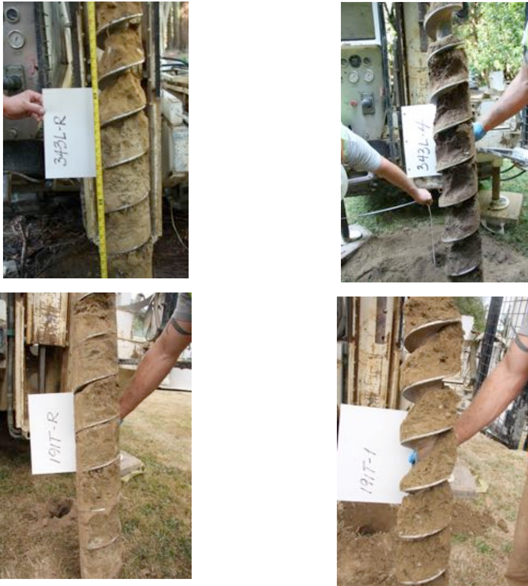
Figure 4.1 Soil photographs during auger drilling.
