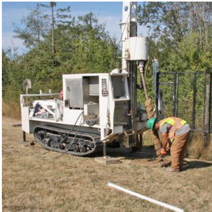
Figure 3.3 Drill rig used for installing the deep monitoring wells.
