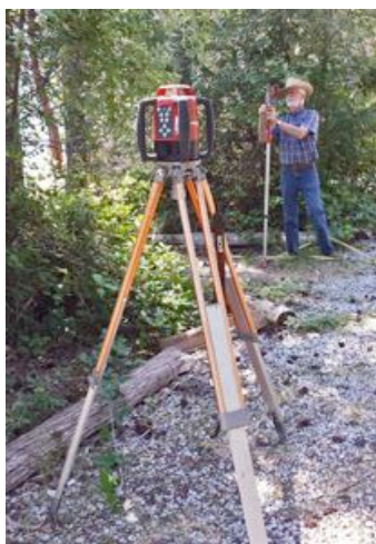
Figure 4.5 Levelling the monitoring wells.
