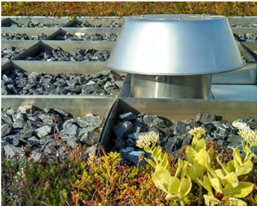
Figure 13 Green-Blue Combination Roof (Capital Region Water Harrisburg, 2017)
