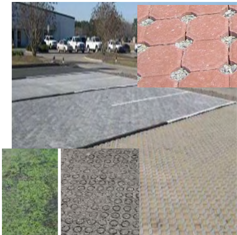
Figure 11 Permeable Pavement Parking Lot (Tetra Tech Inc., 2011)
