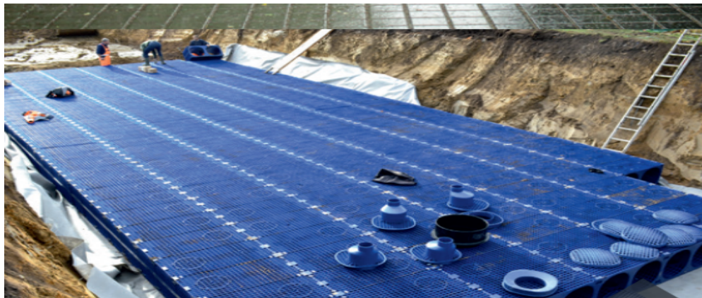
Figure 14 - A soakway designed to prevent water pooling and flooding in parking lots, playfields and other open locations (State of Green, 2015)
