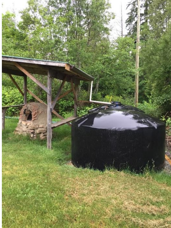
Figure D10. Case study on Phoenix elementary school image taken by Kendra Anderson during site visit on May 30, 2017 to gather further details on RWH systems that exist on SSI. A 2,200 liter tank is filled off the roof of a structure built specifically for the purpose of RWH.
