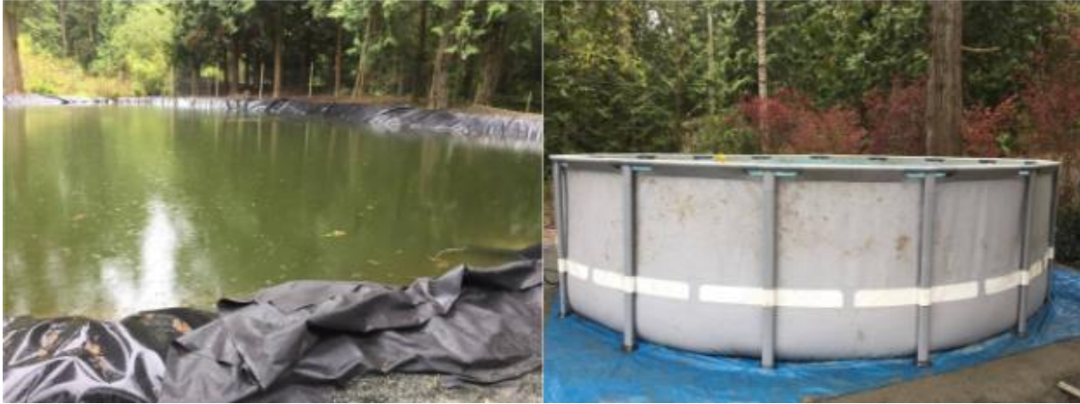
Figure D4. Case study C1 images taken by Kendra Anderson during site visit on April 22, 2017 to gather further details on RWH systems that exist on SSI. Rainwater is collected and stored in the 250,000 gallon lined pond, with the above ground pool used for chlorination and off-gassing for disinfection.
