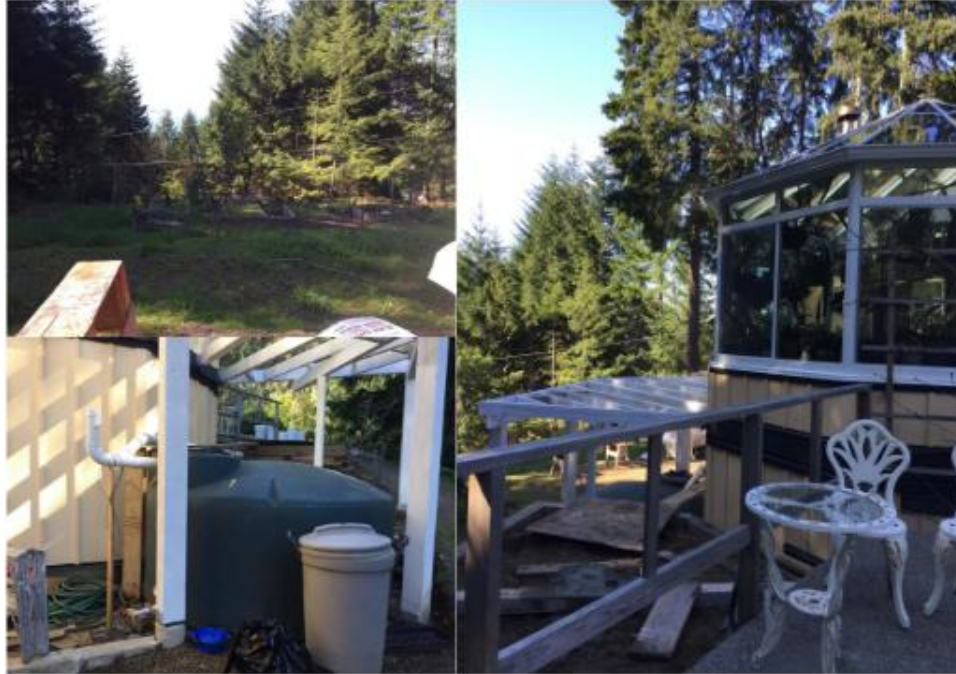
Figure D8. Case study S2 images taken by Kendra Anderson during site visit on April 21, 2017 to gather further details on RWH systems that exist on SSI. Rainwater is collected off the conservatory roof and used on the garden area which is shaded through the afternoon to minimize water use. A 1,100 gallon is used for storage.
