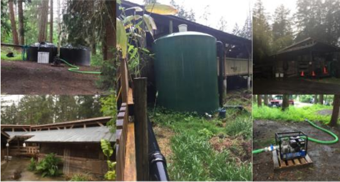
Figure D6. Case study C3 images taken by Kendra Anderson during site visit May 30, 2017 to gather further details on RWH systems that exist on SSI. A 2,100 gallon black cistern is filled from collection off the metal roof and pumped for use in irrigation. The tank was repurposed from previous projects.
